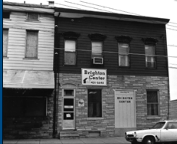
The building on 8th & Central purchased with help from the Guild.
