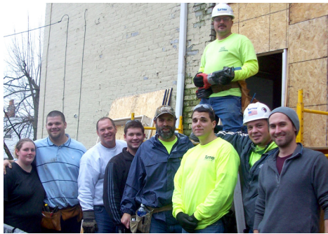
Turner Construction employees volunteer to help a family with home repairs
